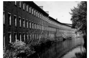
View looking north west at the South Upper Canal Building in the foreground and the North Upper Canal Building in the background. The Upper Canal runs along the east side of the buildings.
